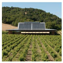
On the Lytton Springs winery's south-facing roof, almost 400 photovoltaic panels supply 75% of the winery's electricity needs over the course of a year. The winery itself is constructed of straw hay bales creating a highly insulated
