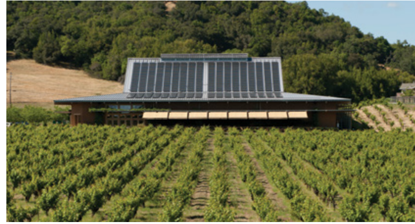
Above: Our solar panels supply a significant portion of the Lytton Springs winery’s electricity needs.
